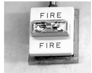
Are visual alarms not more than 50 feet apart and mounted 80 inches above highest floor level or 6 inches below the ceiling, whichever is lower?
